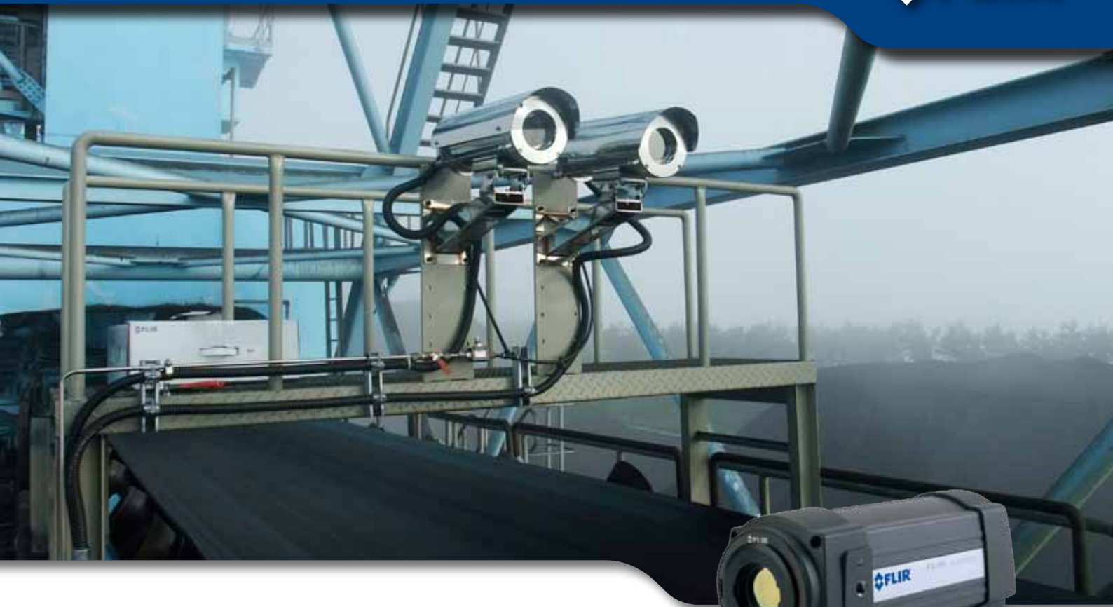
FLIR A310 thermal imaging cameras are mounted in protective housings above the coal transport belts.
